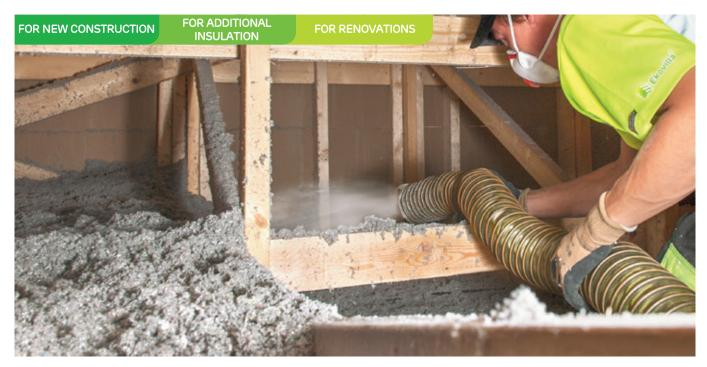
Ekovilla Loose Blown Wool insulation fills every nook and cranny snugly, and the whole layer of insulation planned for the structure is blown in at once. Structural preparation and air-sealing work done before blowing the insulation in is the key to successful insulation and trouble-free installation. Ekovilla is happy to provide instructions beforehand, and will also offer advice on the site, if necessary.
