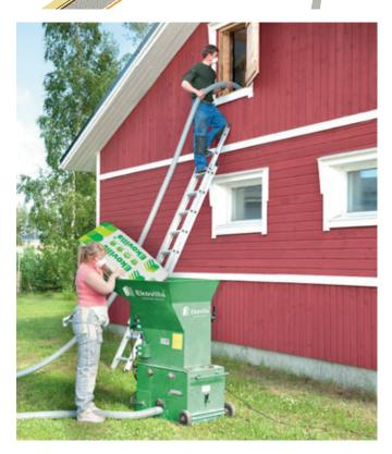
As self-installation, you can blow in insulation to inclined roof cavities, base floors, and walls in addition to the roofing pictured, by using cavity blowing. You can find the instructions on the ekovilla.com website. Depending on the layer of insulation being blown in, flat roofing requires 2 - 3 sacks/m<sup>3</sup>.
